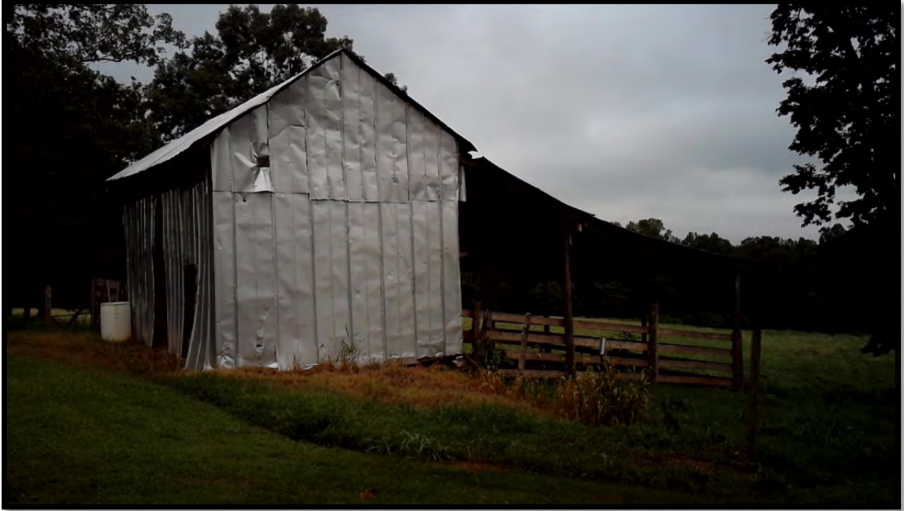
West elevation of livestock and hay barn looking east
