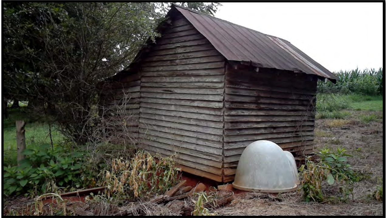
Northwest corner of hog barn looking southeast
