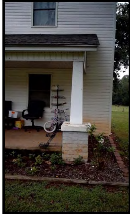
Vinyl over wood columns with brick piers
