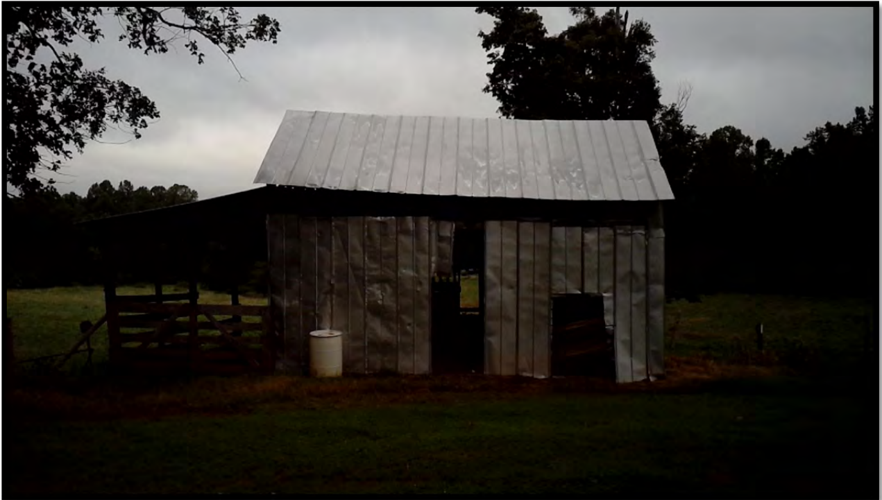
Front (south) elevation of livestock barn, looking north
