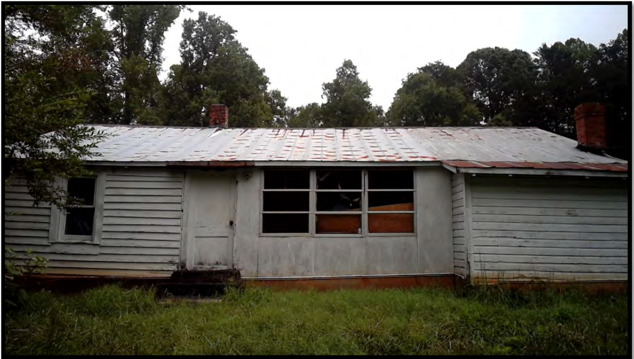
Rear (west) elevation; enclosed rear porch
