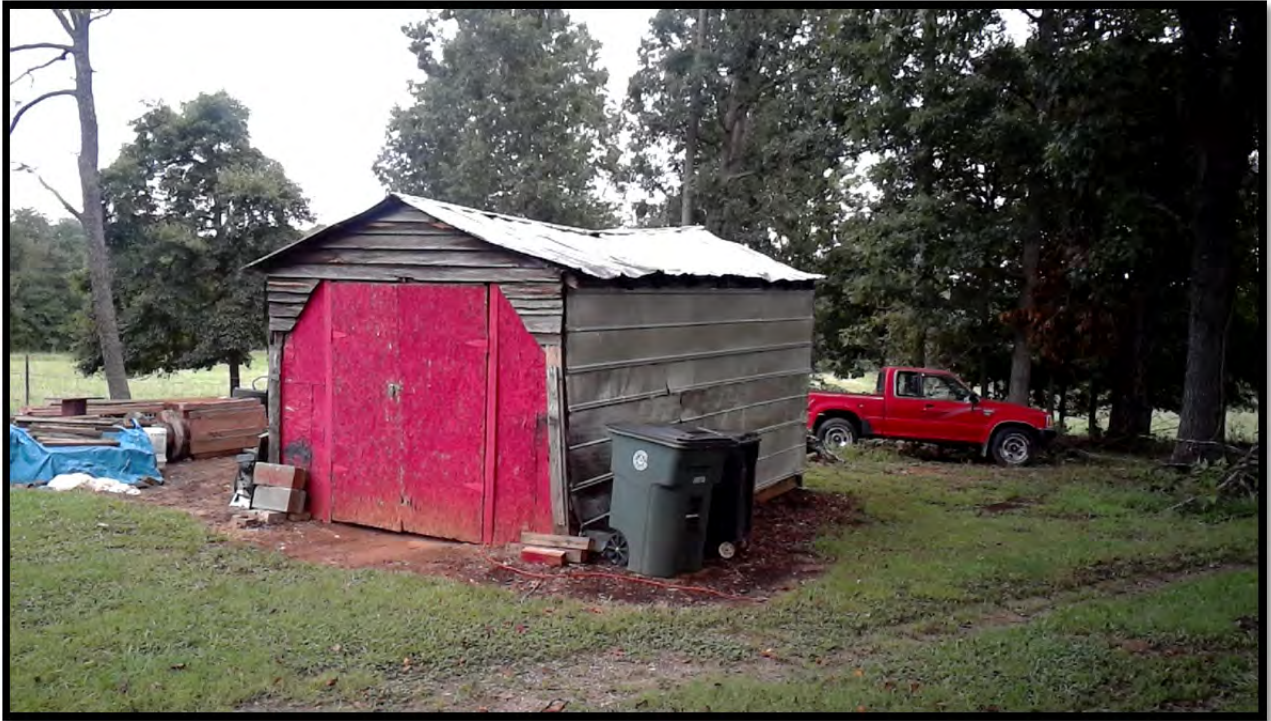
c.1930-40s car shed looking northwest
