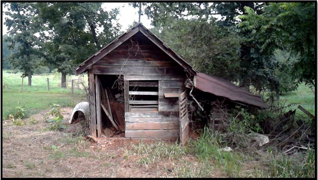
Front of hog barn; looking north
